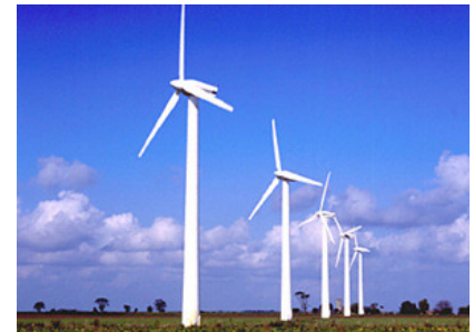
wind power plant
