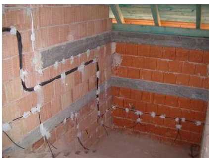
During electrical installation
